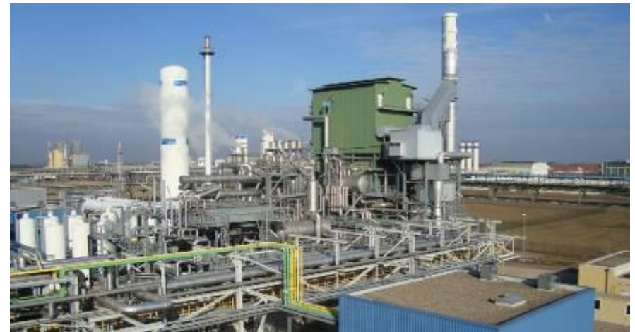
Steamreformer II (35.000 Nm 3 /h hydrogen capacity)
